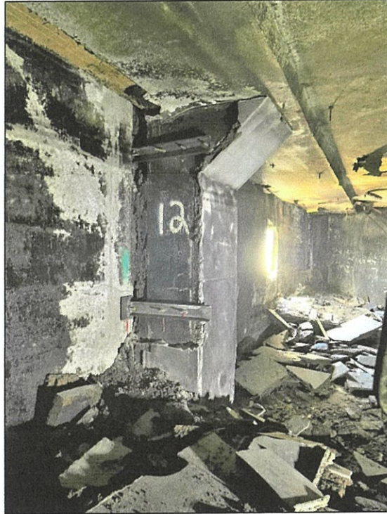
Photograph 15- (10 th floor- wall brackets @ column 12)
