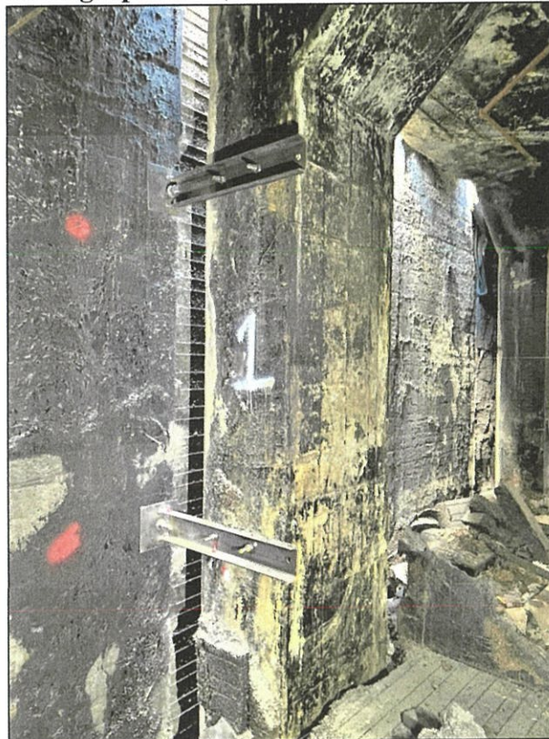
Photograph 12- (11 th floor- wall brackets @ column 1)
