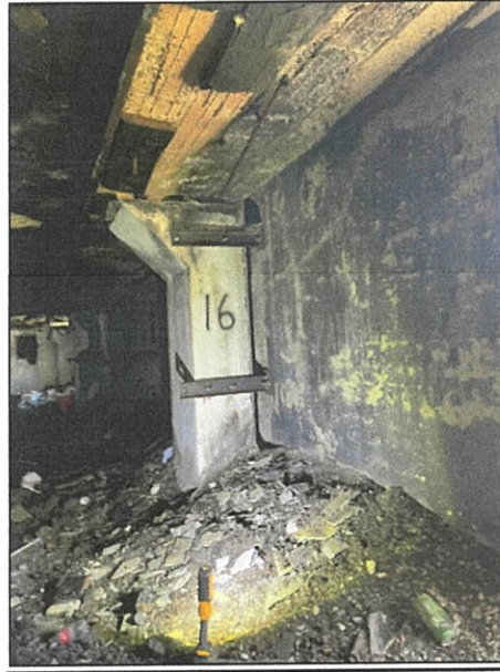
Photograph 17-(9 th floor-wall brackets @ column 16)
