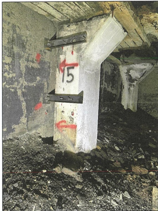
Photograph 16- (9 th floor- wall brackets @ column 15)
