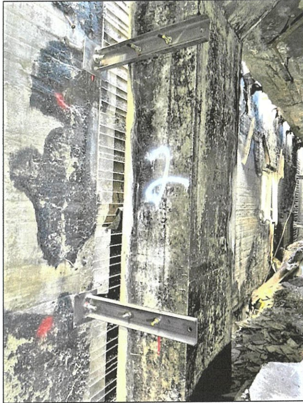
Photograph 13- (11 th floor- wall brackets @ column 2)
