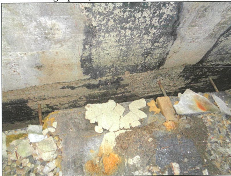
Photograph 10 – (10 th floor level existing wall ties)
