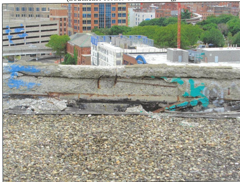
Photograph 5 – July 26 th , 2022 (Southerly roof parapet wall adjacent to the Amtrak tracks)
