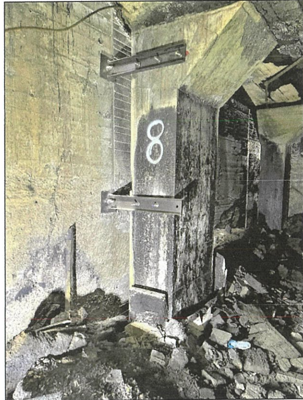
Photograph 14- (10 th floor- wall brackets @ column 8)
